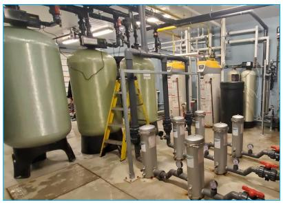
activated carbon, and a bacteriostatic metal alloy to ensure efficient removal of Manganese and Iron, as well as to prevent biological overgrowth. The influent water is chlorinated to aid in the metals removal and continuously regenerate the media's coating, ensuring a very long lifespan.
